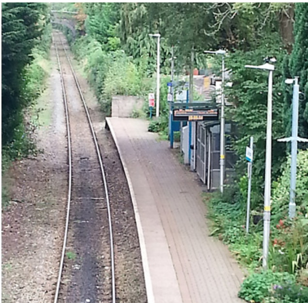
SCMS installed in Wales, UK SCMS Installation in Wales, VK
