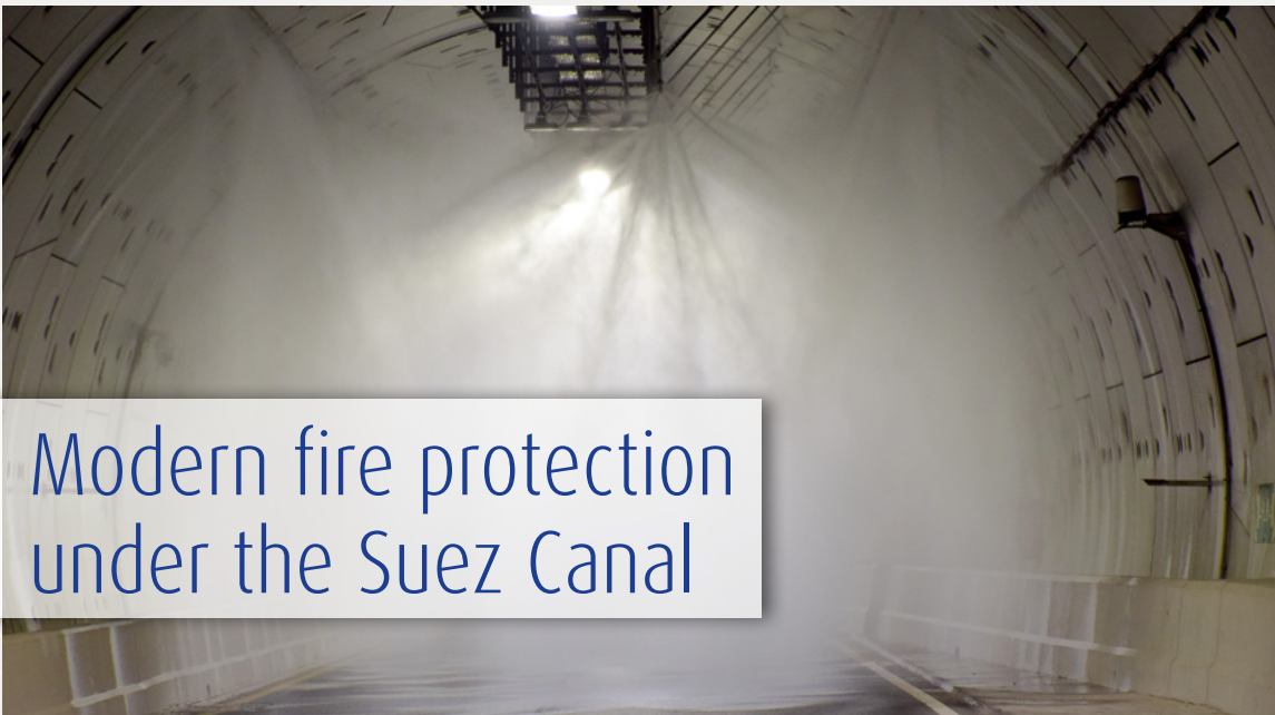
Acceptance test with spray test during commissioning
