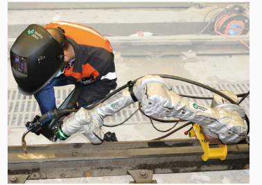
Demonstration on the rails of a customer Photo: Welding Alloys
