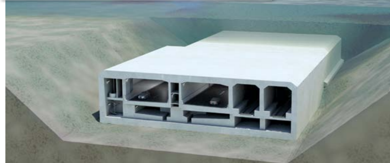
Special element with basement
