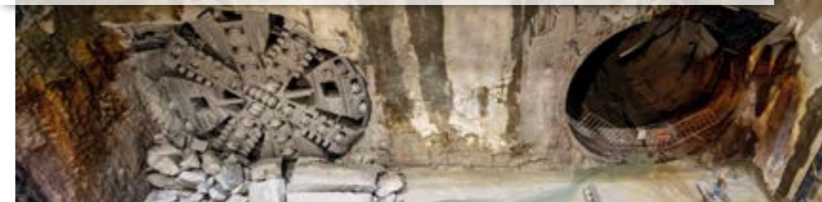
Tunnel breakthrough with a Herrenknecht TBM under Sydney Harbour
