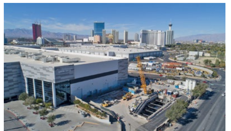
Construction site of the LVCC
